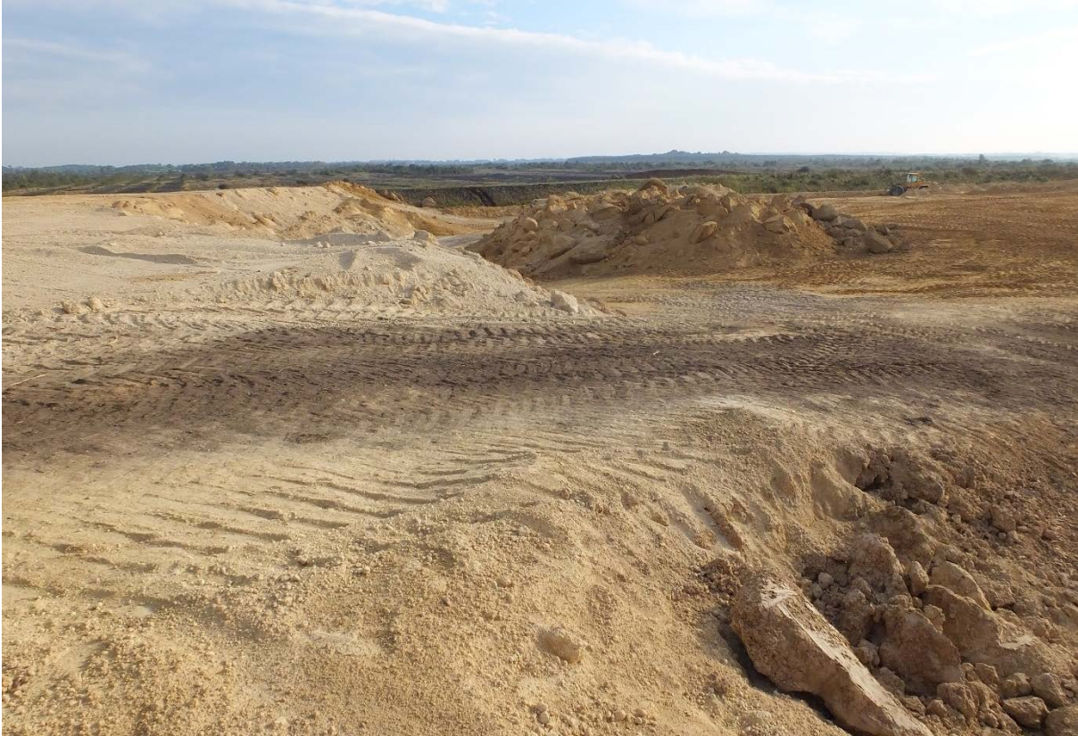
Plate 6.4: Spoil and bare ground (ED2) associated with active ash deposition cell
